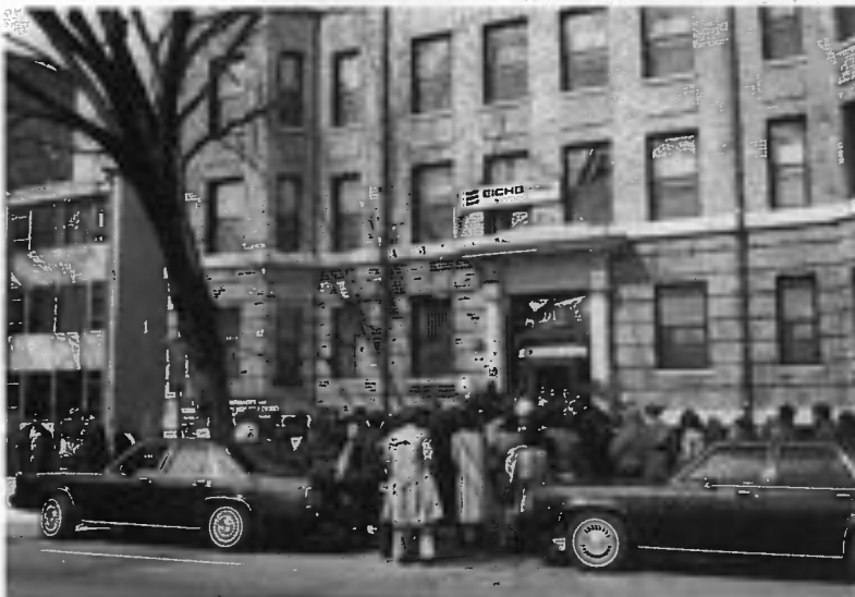
The 919 L Street Cooperative, before and after rehabilitation. Washington Innercity Self-Help Papers , Courtesy, D.C. Community Archives, Washingtoniana Division, DC Public Library
